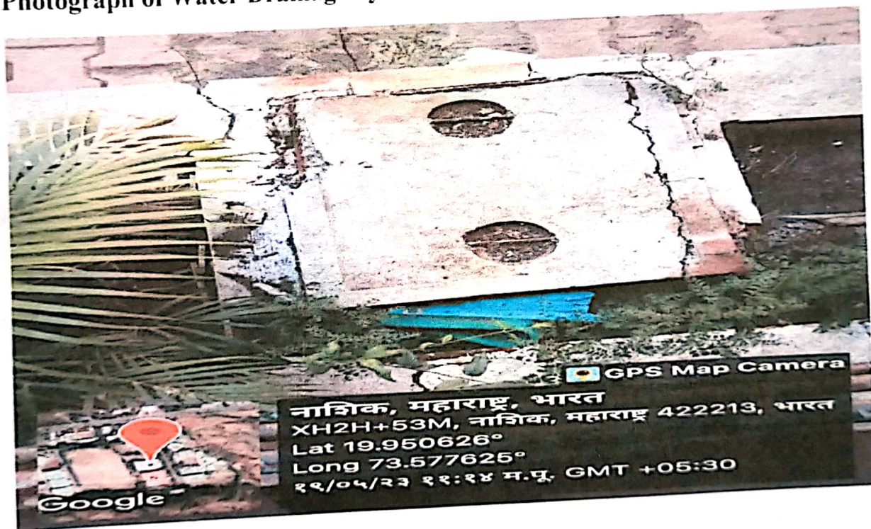
Photograph of Water Drainage Pit
