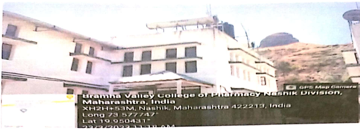
Photograph of Solar Thermal Hot Water System
